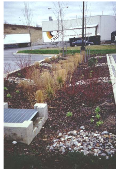
Bioretention System. Photo: Center for Watershed Protection
