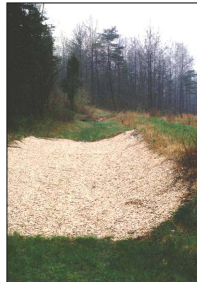
Infiltration trench. Photo: Center for Watershed Protection
